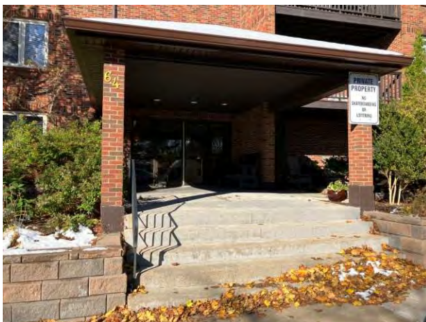
Main entrance concrete slab
