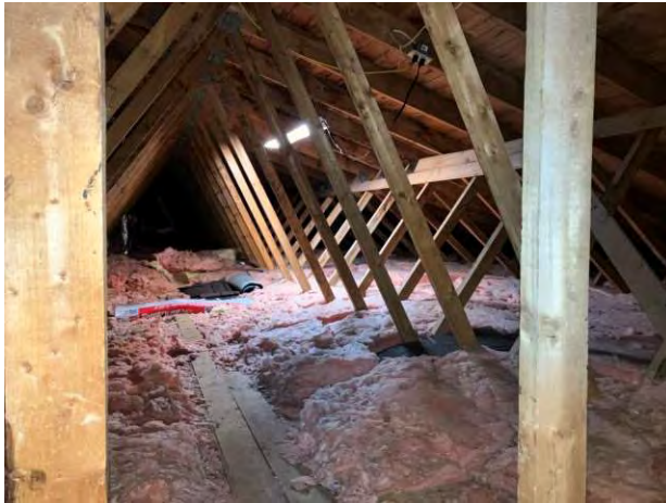
Typical view of attic truss system, lighting, and insulation
