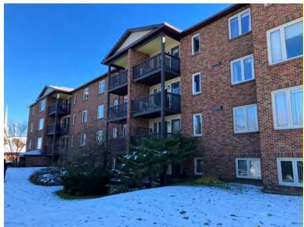
View of typical soft landscaping at west elevation
