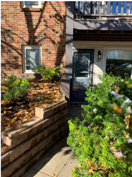
Stone block patio retaining wall at northeast side of property
