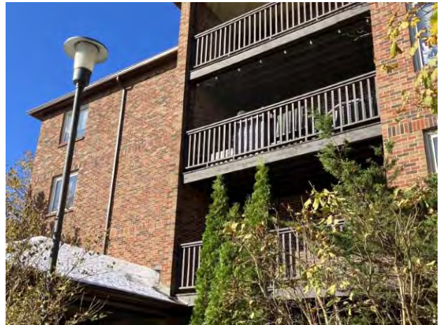
Typical pole lighting
