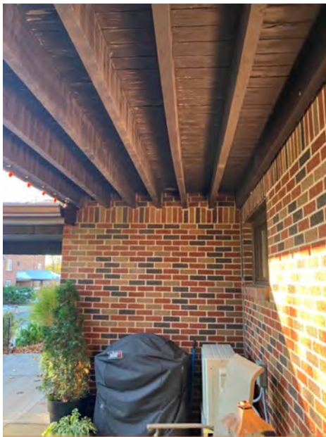
View of underside of balcony
