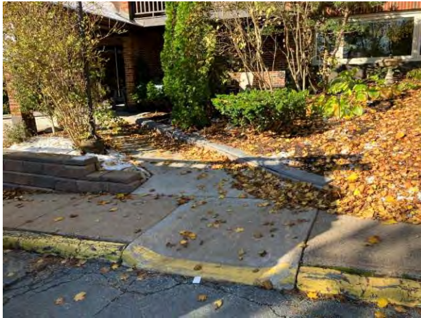
Concrete accessible ramp
