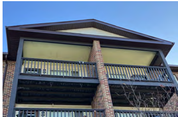
West elevation fascia above balconies
