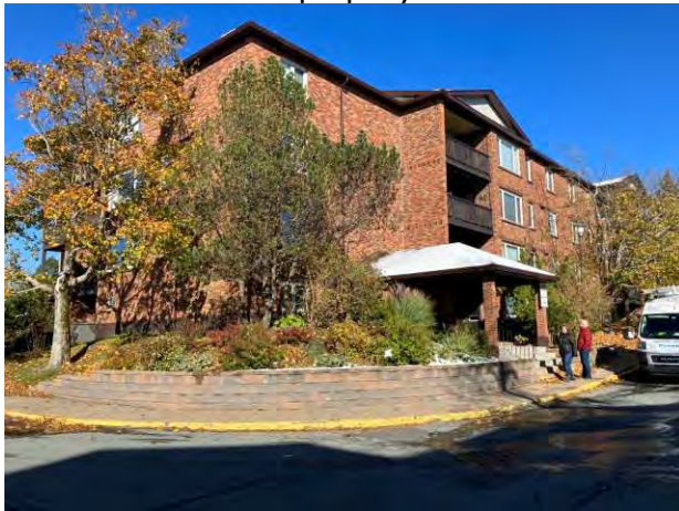
Stone block retaining wall at southeast corner
