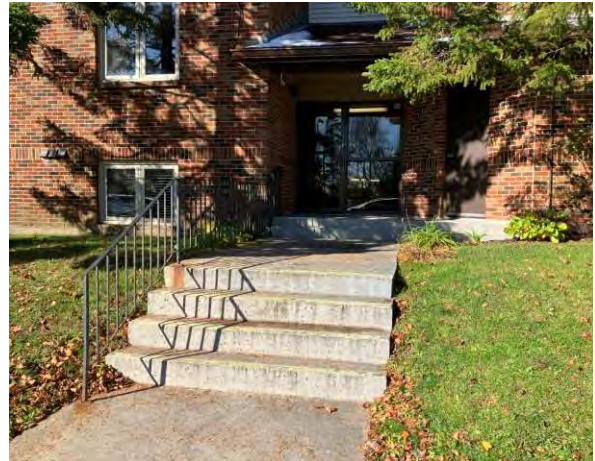
North entrance metal handrail
