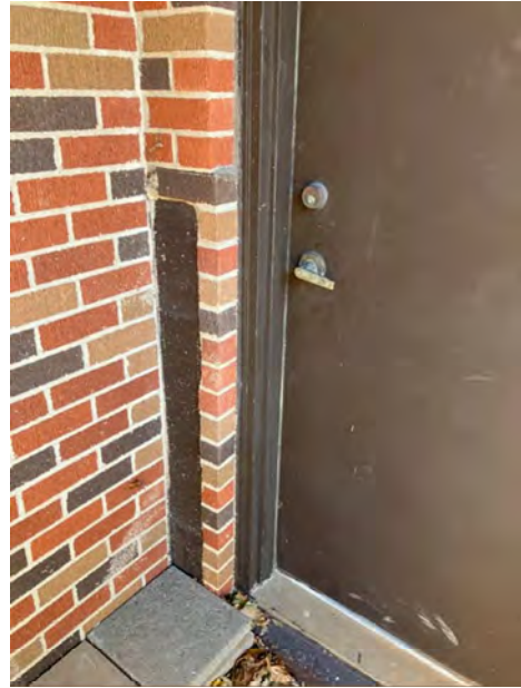
Caulking between brick and metal door frame
