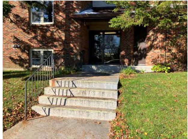
North entrance concrete stairs
