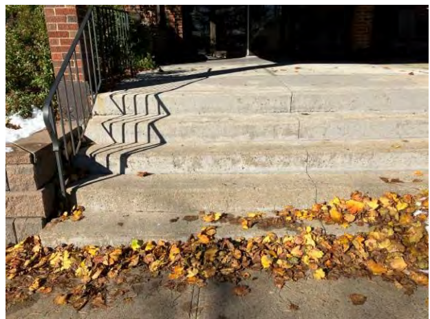
Main entrance concrete stairs
