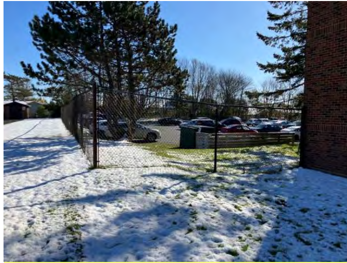
Chain link fencing at north end of property
