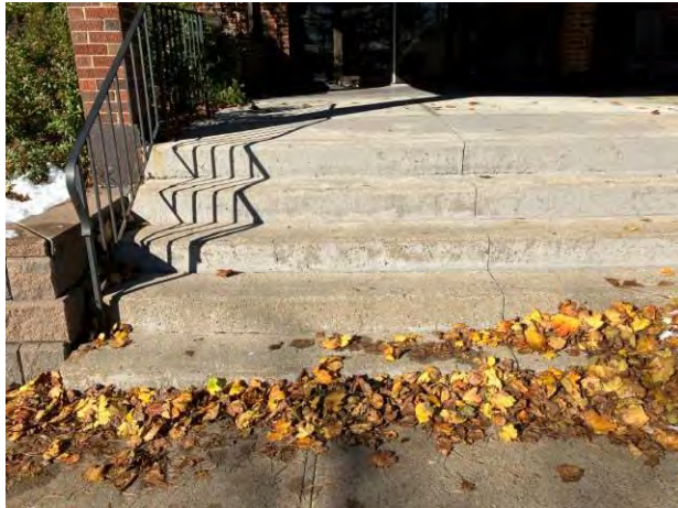
Main entrance metal handrail
