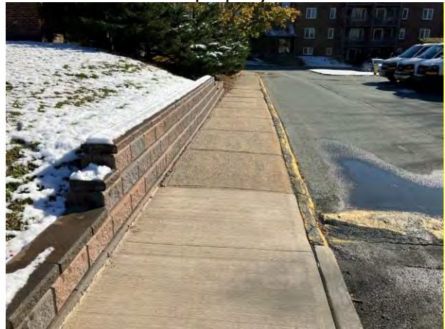
Stone block retaining wall at southwest corner
