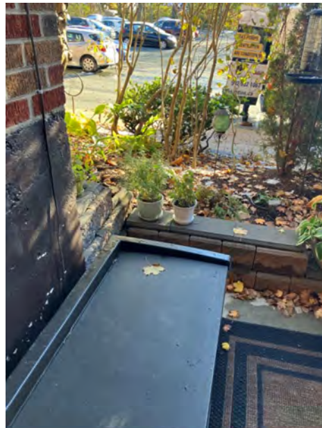
Stone block patio retaining wall at southeast side of property
