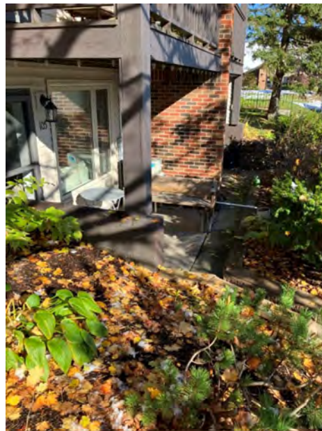
Typical concrete patio at northeast corner
